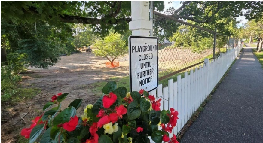
Centerville Recreation Playground Under Construction
