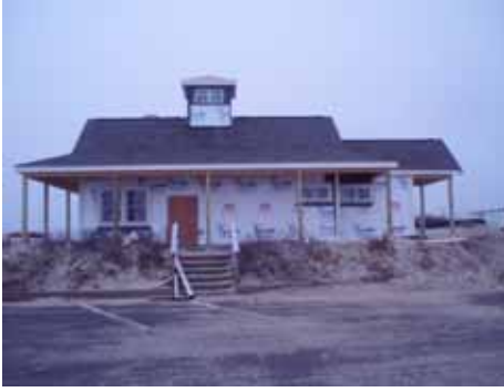
View from the north side. Notice the nice overhangs.
