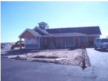
This is the front view of the bathhouse. The siding is up and the roof shingling is complete. The cupola is up. Brass on top of cupola is there.
