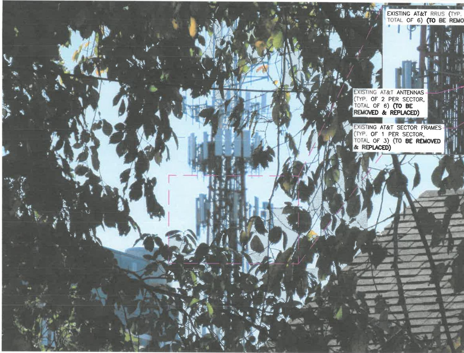
EXISTING AT&T RRUS (TYP. OF 2 PER SECTOR, TOTAL OF 6) (TO BE REMOVED & REPLACED)
